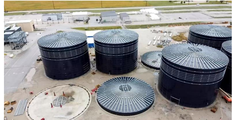
VERBIO plant in North America
